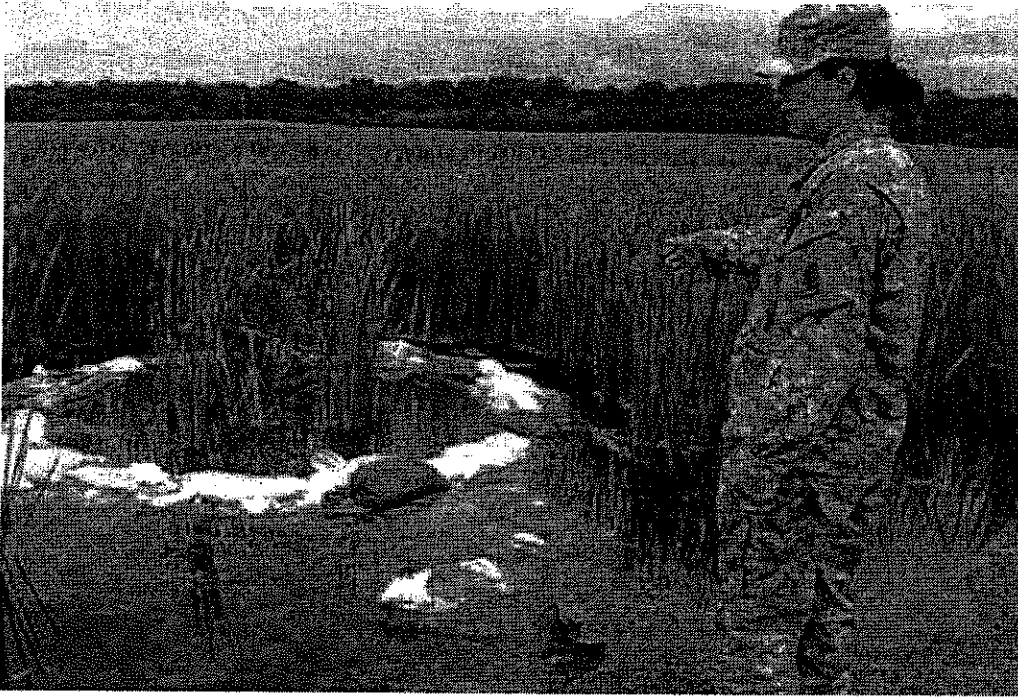
National Guard Sgt. Jillian Kinzer points out a sand boil the patrol has covered and has been monitoring. The boil is just beyond another enormous sand boil that was patched along the levee with gravel. The area is just south of Haworth Park.
